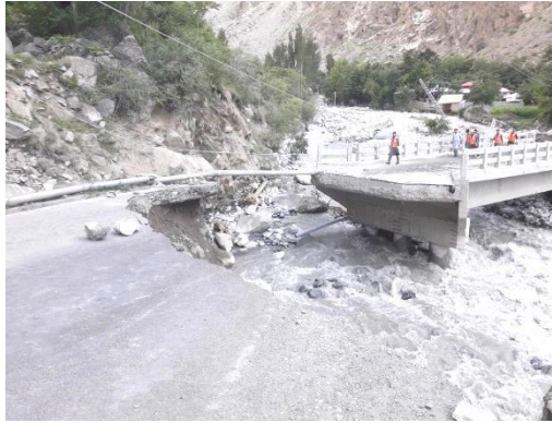
Bridge at Right Bank
