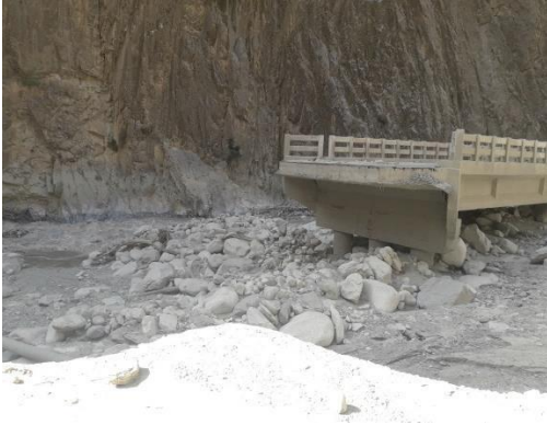
Bridge at Left Bank
